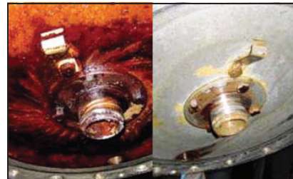
Vessel cover contaminated
